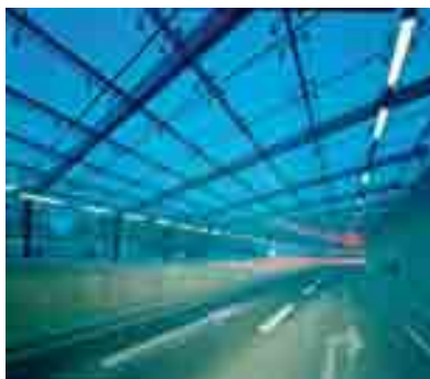
Petuel tunnel in Munich, Germany
